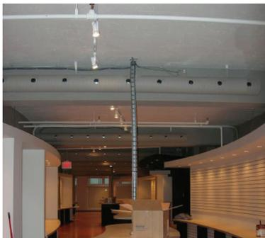
The building owner decided to go with Hi-Velocity equipment so that the ceiling height could be maintained and no structural changes would be needed to the building. Energy Saving Products Ltd. Hi-Velocity System was the ideal choice, the round plenum runs on the ceilings with drilled outlets were easily installed. Using drilled outlets in the plenum was cost effective, and allowed for a fast setup time.
