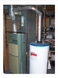
"This is an installation that I performed at a house in Morinville, AB. The furnace was an old Flame Master along with a 30 gallon John Wood hot water heater. I met the homeowner at a local renovation show and showed him the benefits of installing a "Combo System" using a 75 gallon hot water heater and an Energy Saving Products Lo-Velocity Air Handler"
