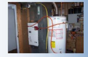
"This also reduces the total BTUH firing capacity of the home by 45%. The original furnace input was 110,000 BTUH and the original hot water heater was 33,000 BTUH. This gave us a total of 143,000 BTUH. By installing the Lo-Velocity and hot water heater combo system the total capacity was reduced down to 75,000 BTUH."
