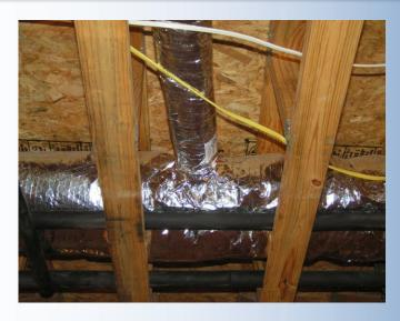
The two inch ductwork results in less custom sheet metal work, minimizing waste and provides the flexibility for complex architectural designs. The high moisture removal of the Hi-Velocity Systems will remove up to 30 percent more humidity from the air, providing greater comfort while eliminating the cold clammy feeling that can exist with conventional systems.
