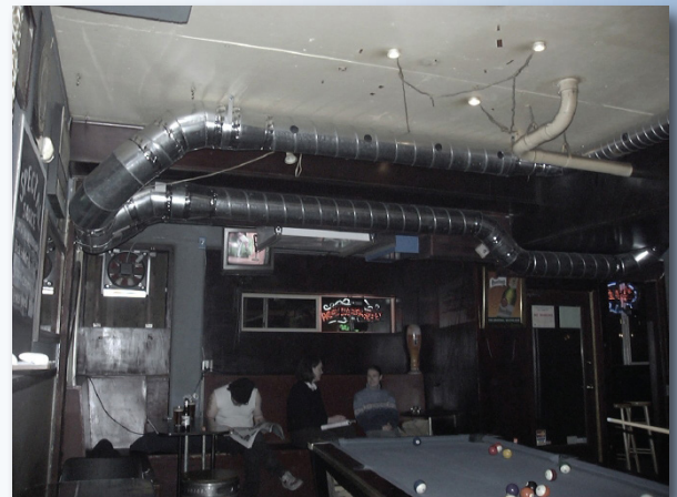
Exposed Duct with Drilled Outlets in Games Room
