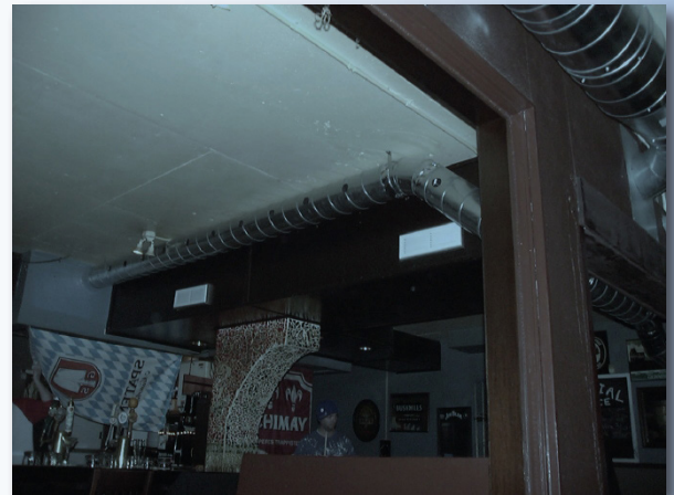
Exposed Duct with Drilled Outlets
