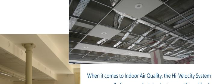
when it comes to Indoor Air Quality, the Hi-Velocity System can answer all of your needs. Introducing conditioned fresh air from a HRV/ERV or simply bringing a fresh air supply into the return air of the system can make your office or commercial space much more comfortable.
